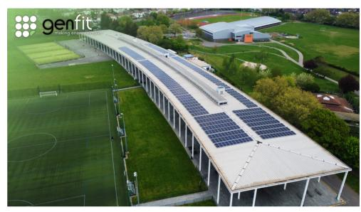
300 kWp 659 panels 263 MWh p.a.
